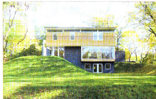
Above: The home's exterior is composed of charcoal-colored concrete block on the first level and ochre fiber cement panels on the second level. This backyard view shows the "land pier" or hill, that was built to create a terrace off the kitchen. Steps lead down to the lower-level walk-out.
