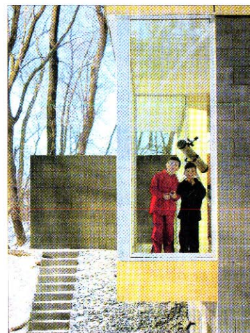
Above: The home's exterior is composed of charcoal-colored concrete block on the first level and ochre fiber cement panels on the second level. This backyard view shows the "land pier" or hill, that was built to create a terrace off the kitchen. Steps lead down to the lower-level walk-out.
